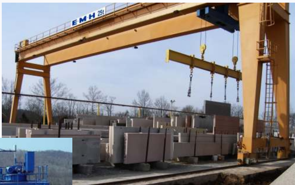
A 25 ton, 120 foot gantry (above) positions architectural concrete panels from production to storage..
