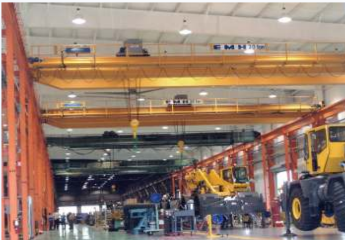
30-ton cranes with walkways are used in the production process at a Pennsylvania manufacturer of mobile cranes.
