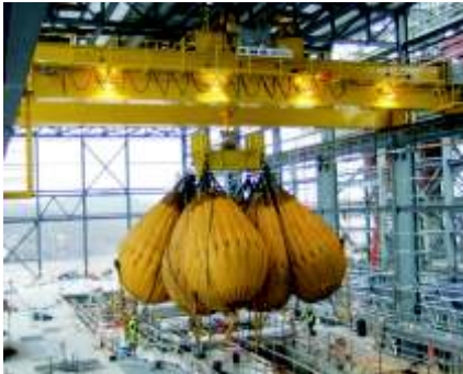
Overhead Bridge Cranes
