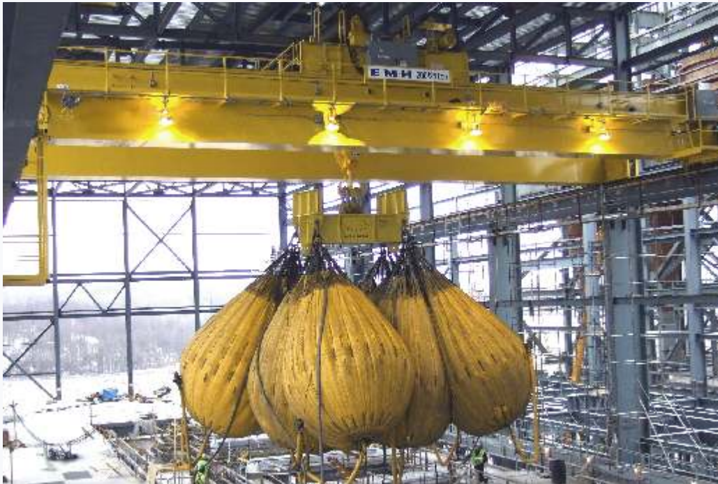
A 250/50 ton engineered crane undergoes load testing at a power plant.
