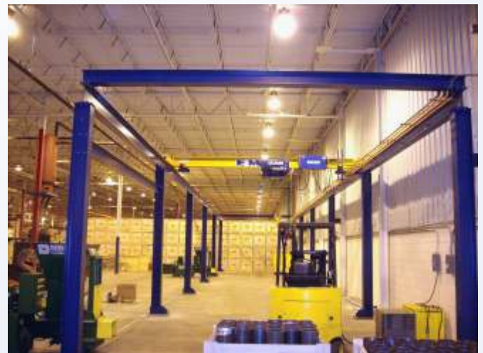
A modified NOMAD with one side tied back to the building structure.
